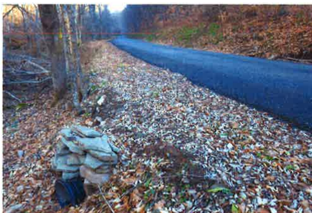
The same section of road during the final inspection. Surface stabilization of the cart way combined with pipes cut fluvial erosion.
