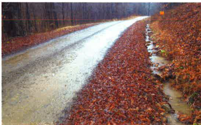
Deering Run Road in Summit Township during the pre-application meeting. Note the substantial volume of sediment laden flow.
