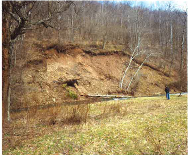
A massive persistent erosion sloth on the South Branch of the Sinnemahoning is exacerbated by stream meander. The approximately $150,000 face lift will use soil nails to hold concrete stabilizer in order to prevent the cliff from further collapse. To allow such a collapse would result in a complete loss of the road located on the precipice.
