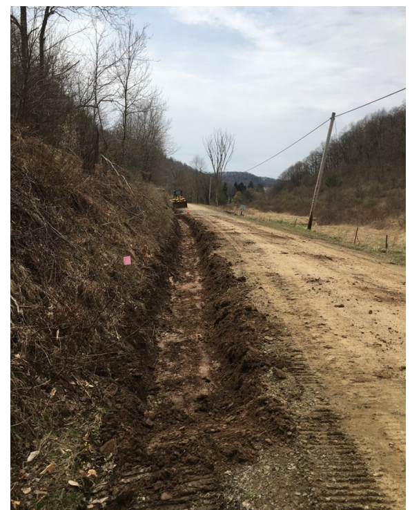
Right: French drain installation on S. Dry Run road project to prevent water in saturated ditch from leaching into road base
