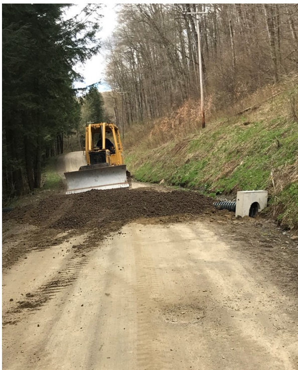
Left: Backfilling shallow cross pipe installation on Southwoods Road project. Completed 30 cross pipe installations on project
