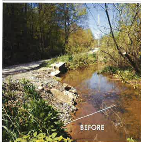
Before this project, the road profile is significantly lower than the stream profile, easily leading to stream and drivability problems. The road was raised over 4 feet, and mudsill cribbing was added where the difference was most severe. Other in stream structures included cross vanes (bottom R) and new DSA was laid on the 750' of project length (top R)
