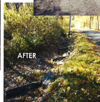
Before this project, the road profile is significantly lower than the stream profile, easily leading to stream and drivability problems. The road was raised over 4 feet, and mudsill cribbing was added where the difference was most severe. Other in stream structures included cross vanes (bottom R) and new DSA was laid on the 750' of project length (top R)
