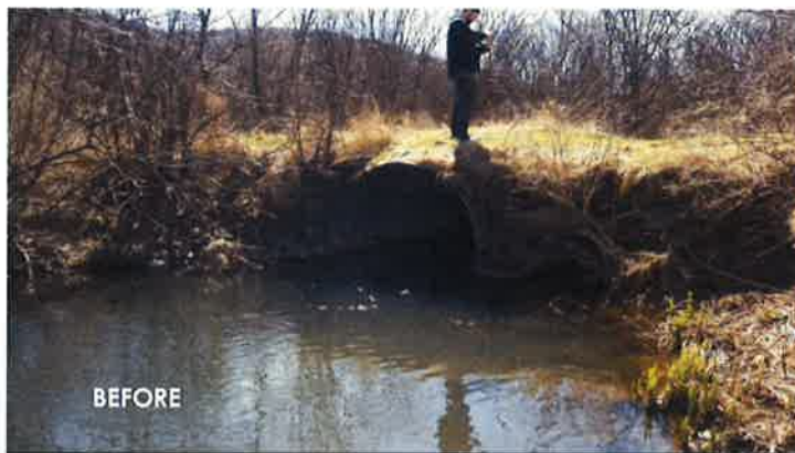
Before the completion of this pilot project, native trout could not access the upper reaches of Ludington Run. Poor drainage fouled the headwaters tributary of the Genesee River with sedimentation and challenged both PennDOT and Bingham Township. The site was chosen as a launch point for the "Potter County Water Quality Protection and Education Initiative."
