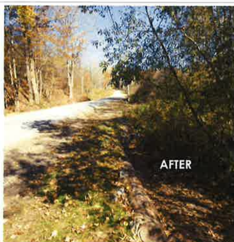
Before this project, the road profile is significantly lower than the stream profile, easily leading to stream and drivability problems. The road was raised over 4 feet, and mudsill cribbing was added where the difference was most severe. Other in stream structures included cross vanes (bottom R) and new DSA was laid on the 750' of project length (top R)
