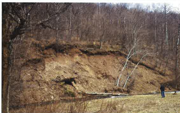
Above, Glenn Dunn II, Resource Conservationist, assisting at a 2017 DGR Southwoods Road project site. Erosion from the hillside deposited directly to the stream below. The resulting project included DGR funding towards soil pinning, new road base and top coat of driving surface aggregate, and installment of a guard rail.
