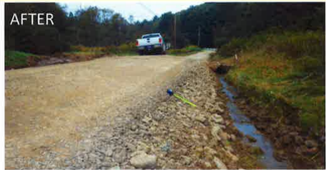
The same road after construction was finished. Base build and cross pipes greatly improved drainage
