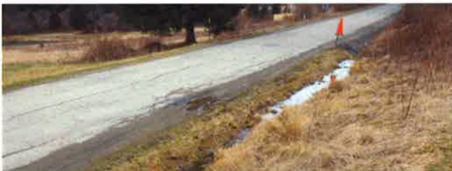
Clara Township-Clara Road LVR: Water in ditches leading to saturated road base, potholes, and road cracking
