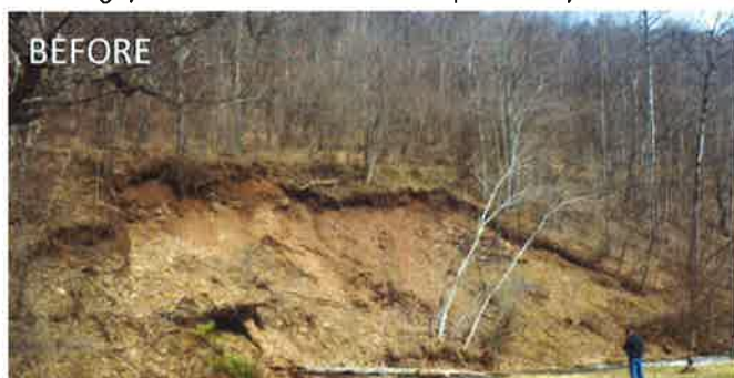
With slope stabilization, streambank stabilization, new guide rail, and a fresh application of DSA, this section of road was much improved. Above, the stream side view of the large slough is pictured before and after the project's completion
