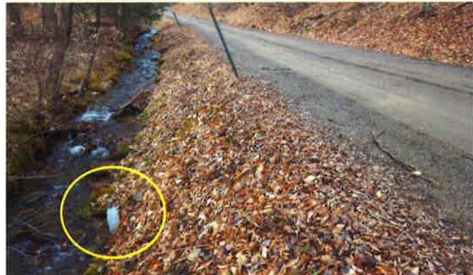
Zoerb Hollow Road in Abbott Township. Note that the underdrain Pipe outlets directly to stream
