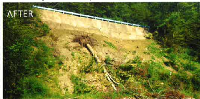
With slope stabilization, streambank stabilization, new guide rail, and a fresh application of DSA, this section of road was much improved. Above, the stream side view of the large slough is pictured before and after the project's completion
