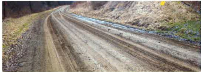
Eulalia Township-Sheldon Hollow Road: Poor road material, in need of base build and drainage.
