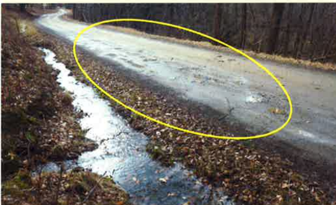
Old Shovel Road in Eulalia Township. Like the site above^ water in ditches leading to saturated road base and potholes
